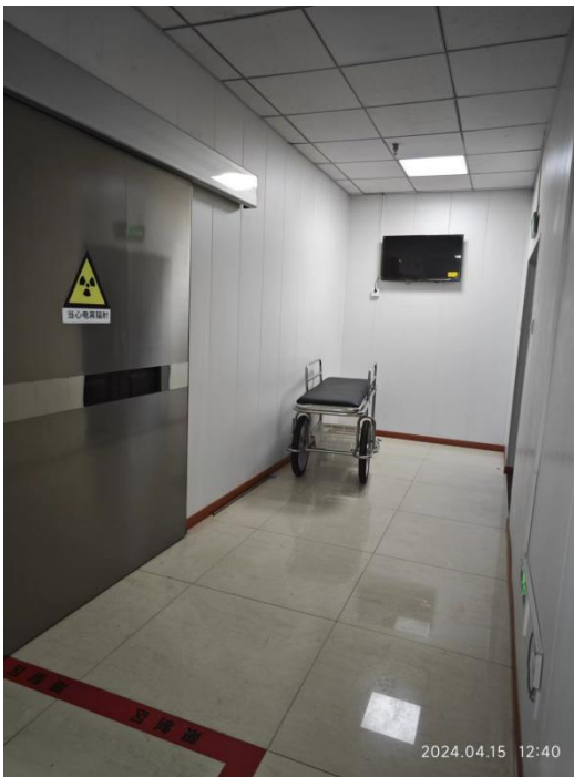
DSA 机房西侧缓冲区
