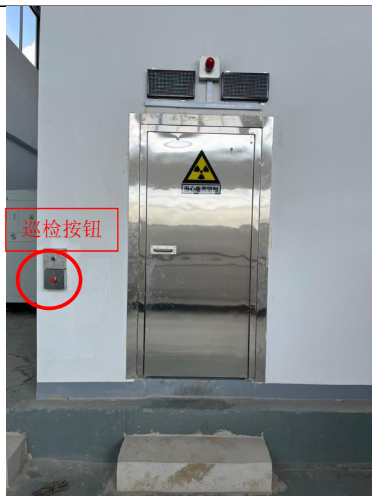
1#加速器机房主机室门口巡检按钮
