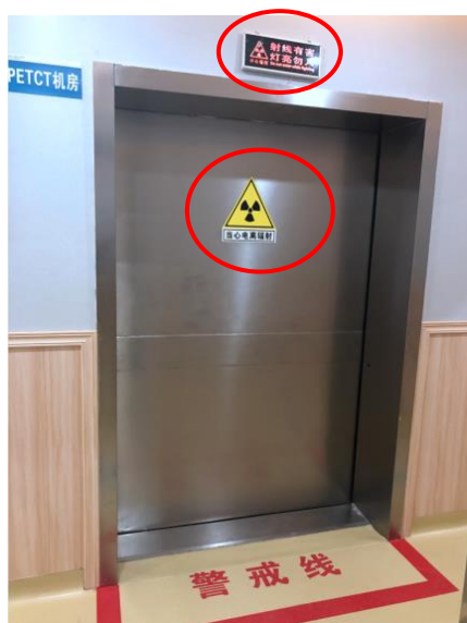
PET/CT 机房防护门
